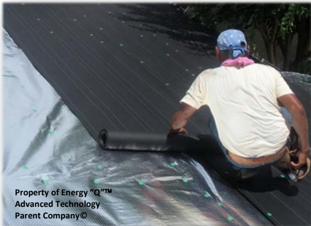
Above: Energy "Q"™. Under Tar Paper
